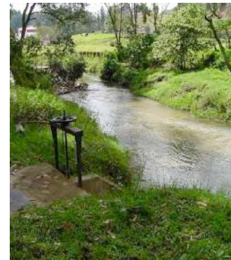
The outlet of treated water into La Mosca creek
