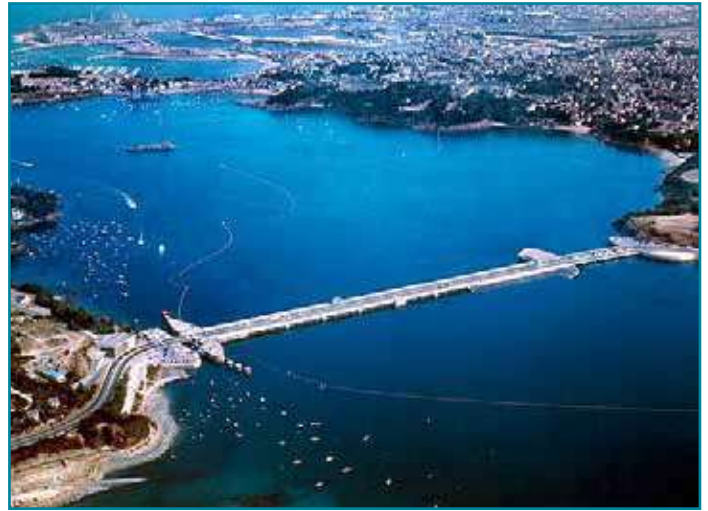
Figure 6. 240 MW ocean power plant La Rance, France
