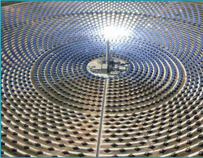
Figure 4. The Gemasolar concentrated solar power plant. Central tower. Seville, Spain
