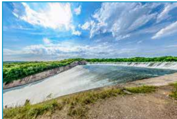
Hydroelectric power station Sanalona, Sinaloa.
