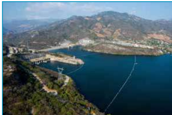
Hydroelectric power station Chicoasén, Chiapas.
