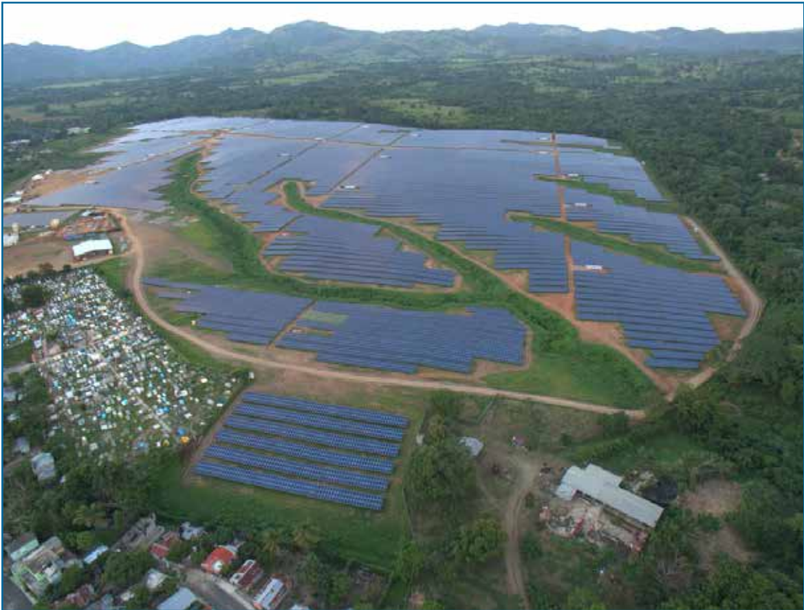
Monte Plata Solar farm. Capacity 30 mW
