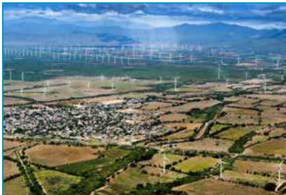
Wind power plant in La Ventosa, Oaxaca.
