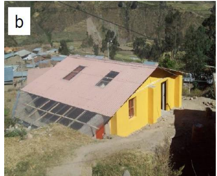
Solar houses in Peru Source: CER –Uni, Lima
