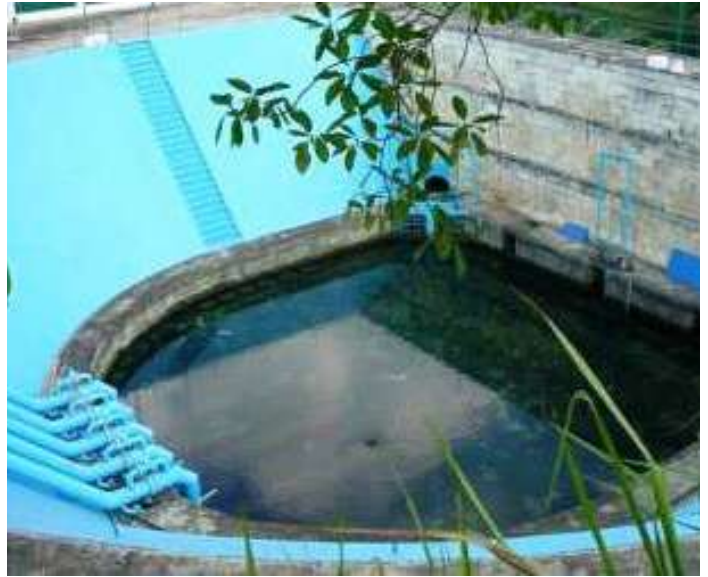
Figure 9. Vento Springs water intake today
