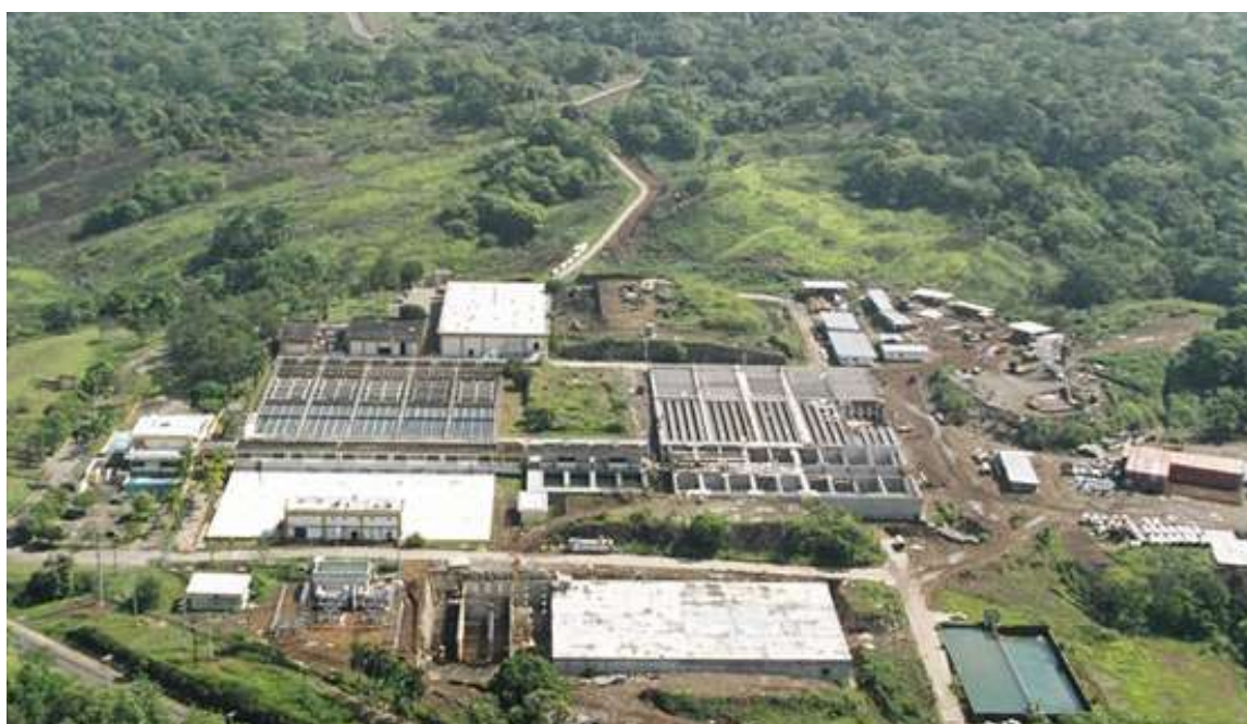
Figure 4. Chilibre water treatment plant with a capacity of 250 MGD, the largest in Panama
