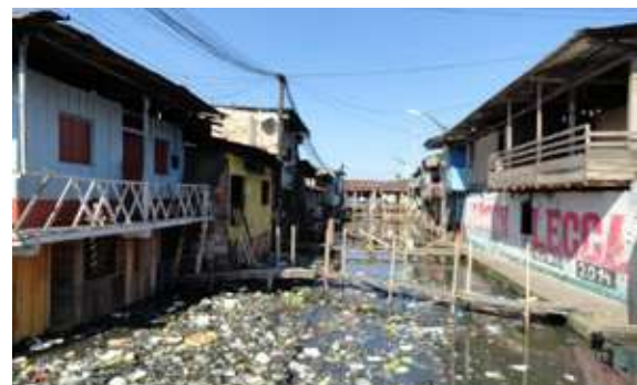
Figure 17. Iquitos, sewers in the neighborhood of Belén
