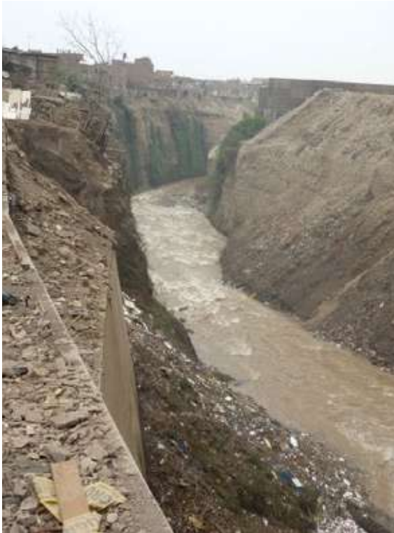
Figure 12. Urban Canyon formed by the degradation of the Rímac Riverbed downstream of Puente del Ejército
